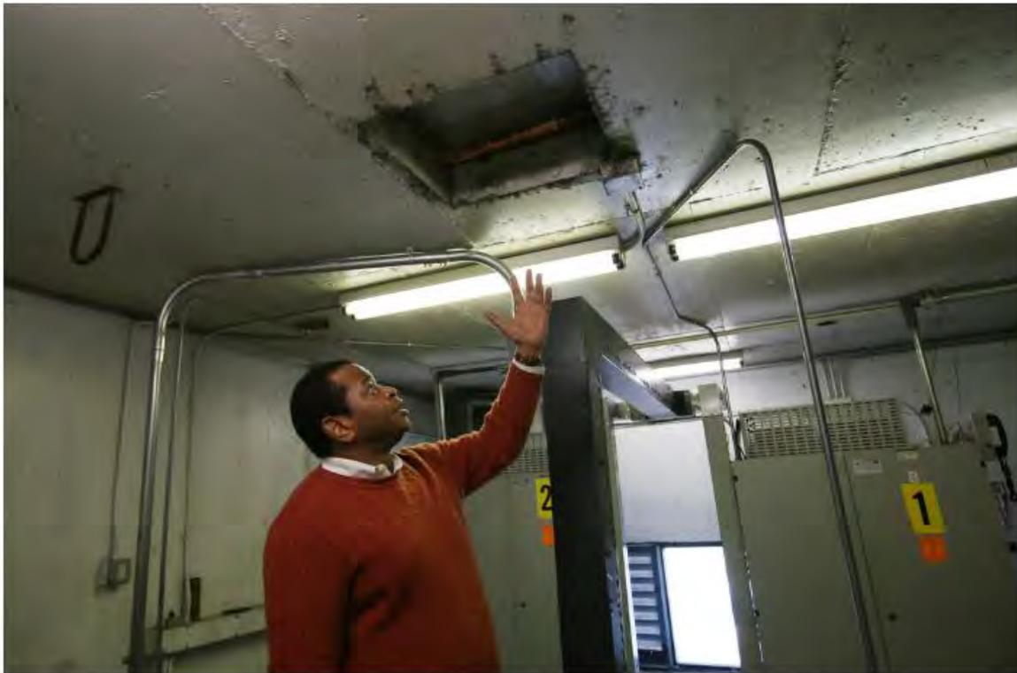
David Davenport, principal of Urban Greenfit, and a hole that had been closed above an elevator shaft. Sealing such cracks and holes, he said, "is critical because the biggest problem is air leakage from buildings."
